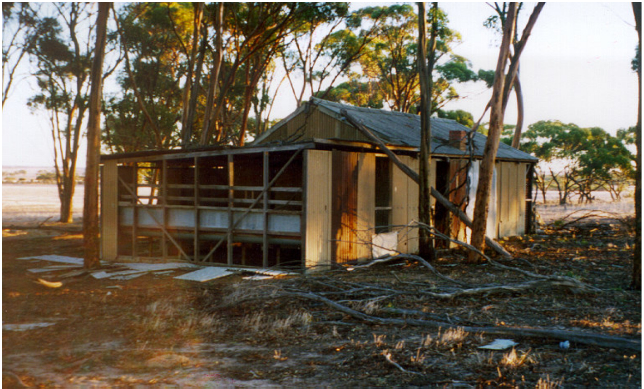
Ablution and laundry building, Ardath Ammunition Depot, Shire of Bruce Rock Photo: B Bridges / H Birch
