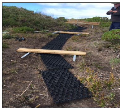
Track P:ads and steps set out on site
