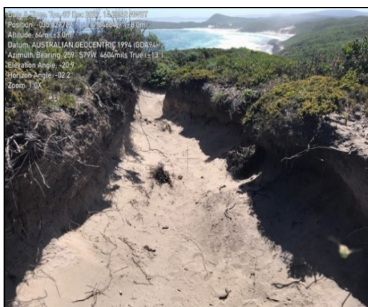
Eroded & damaged steps Peaceful Bay
